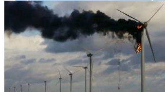
Wind turbine collapse
